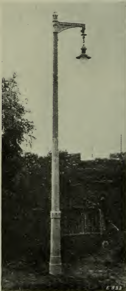
FIG. 7. CONCRETE LAMP STANDARD.
